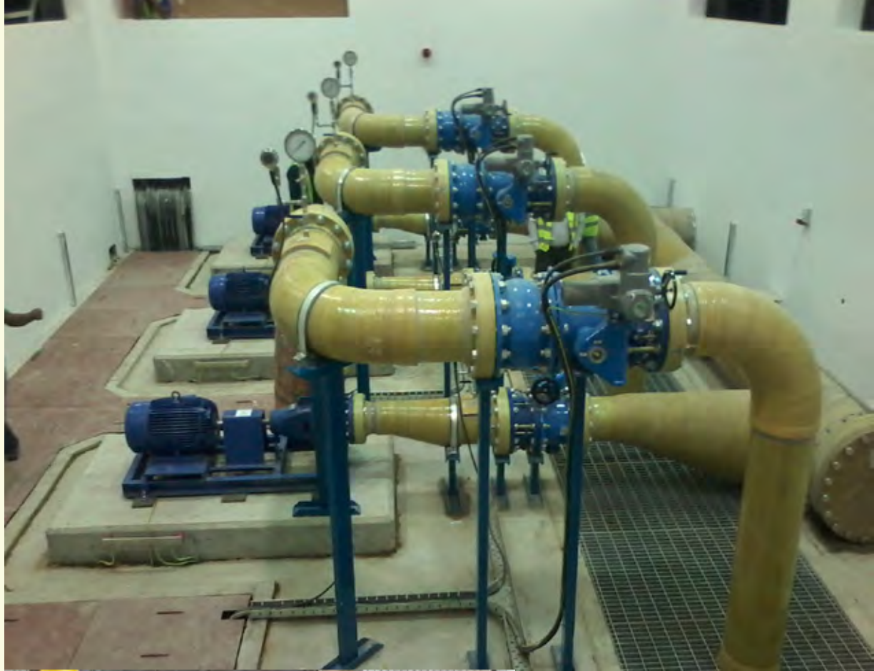
▲ INSIDE THE PUMPHOUSE Inside the pump-house that drives the water towards the service reservoir. The whole system operates automatically using SCADA.
