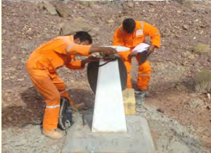
▲ VERIFICATION AND CHECKING Verifying and checking the final survey copper stud inserted into the concrete fulcrum.
