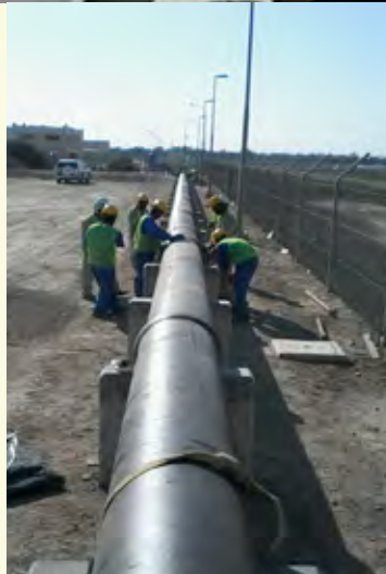
◀ PIPELINES CORRIDOR Above ground pipeline. The pipes' route follows a corridor and goes into the ground and over bridges to avoid congested areas.
