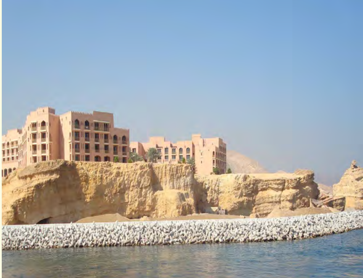
▲ REVETMENT AL HOSN HOTEL Six star hotel “Al Hosn” overlooking the turtle beach area. The revetment protects the weathered and weak cliffs but leaves access to a sandy area for green turtles to come and hatch on the beach.
